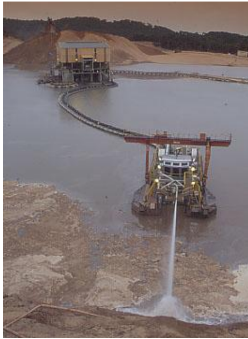
Figure 2: Dredging operation at RBM (Anthony Bannister)
