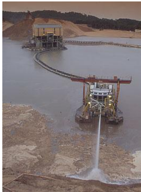
Figure 2: Dredging operation at RBM (Anthony Bannister)
