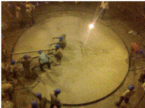
**Figure 6:** Pouring of Levelling castable
