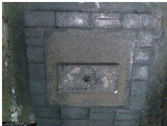
**Figure 9:** Tap block and surrounding bricks inside steel flange as see from outside of furnace
