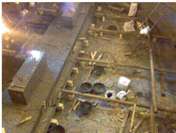
**Figure 7:** GradeD™ carbon block in hearth showing proper jacking by means of jacks and wooden poles
