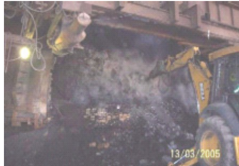
Figure 6: Furnace digging in progress
