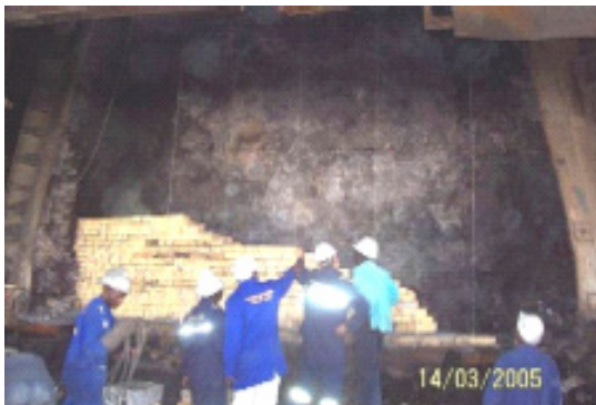
Figure 10: Initial stage of Refractory Installation
