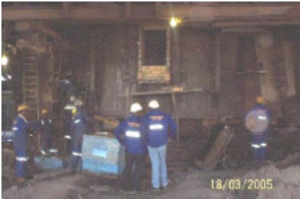
Figure 12: Complete Refractory and Shell Installation
