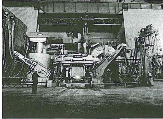
Figure 3, the Twin Electrode DC EAF at HYLSA
