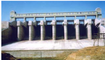
Figure.4 The Gangnan Reservoir in Hebei Province built by steel slag cement
