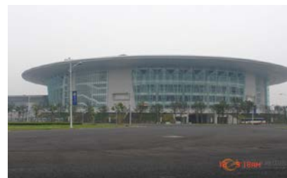
Figure.10 Wuhan Gymnasium built by steel slag concrete
