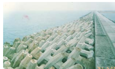
Figure.7 Wave attenuation frame built by steel slag cement
