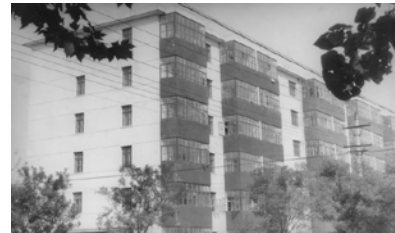
Figure.5 the Residential building built by steel slag cement
