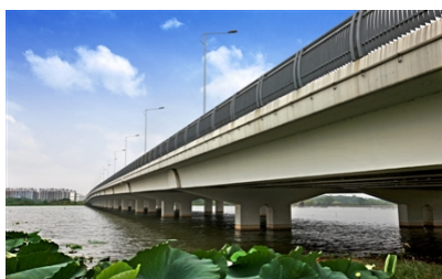
Figure.9 Nantaizi Lake Bridge built by steel slag concrete
