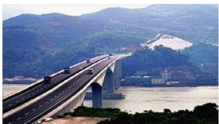
Figure.8 Xiabaishi Bridge built by steel slag concrete
