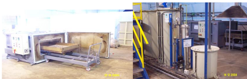
Figure 3: Overview of industrial pilot plant and cell.
