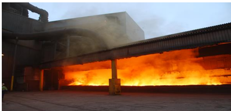
Figure 1: Casting beds showing fume escape from under extraction hood and roof.
