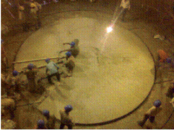
Figure 6: Pouring of Levelling castable
