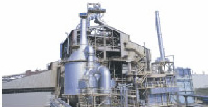
Figure 1: View of the SF at Mizushima Ferroalloy Co., Ltd.
